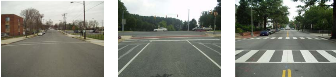
Visibility of various types of crosswalk markings: the high-visibility markings shown in the photo to the right are the easiest for motorists to see
