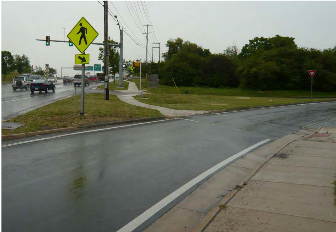
Sidewalks are present on this section of Millwood Avenue with standard pedestrian ramps.
