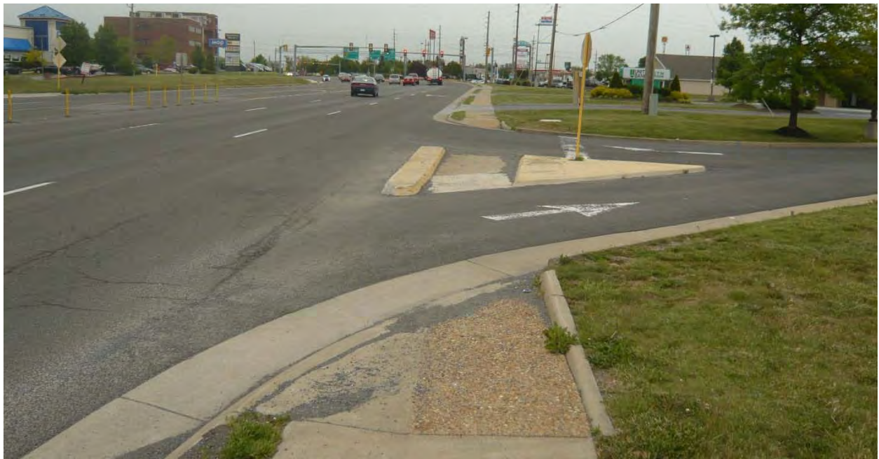
This picture shows the Entrance/Exit to the Costco. Notice the Exit is right only. Delineators are used to prevent lefts. The picture shows that some of the Delineators have been damaged or removed.
