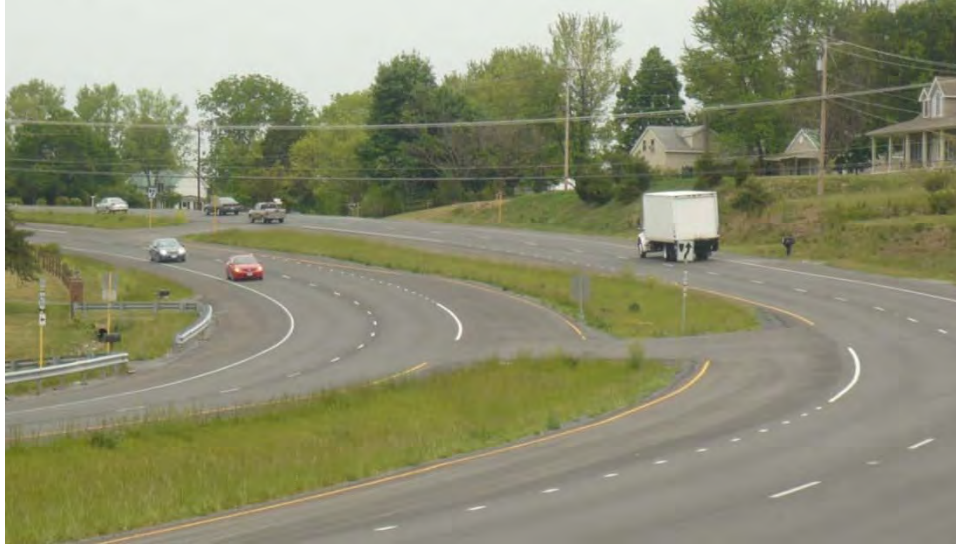
Figure 2-9: Example of Median Crossover Not Meeting VDOT Regulation
