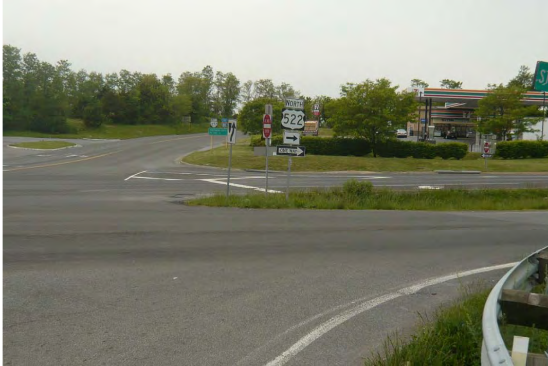
Facing northwest at the traffic signal at the intersection of US 522 and Lord Fairfax Hwy (US 340). There may be clearzone issues with these signs.
