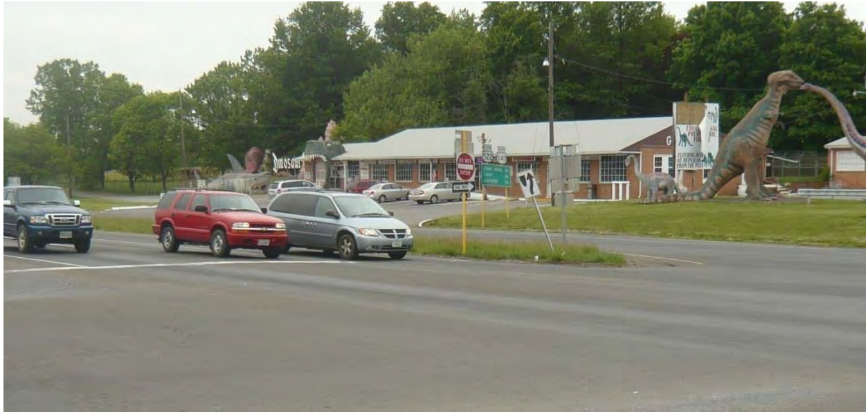
Another picture facing southwest at the traffic signal at the intersection of US 522 and Lord Fairfax Hwy (US 340). There may be clearzone issues with these signs.
