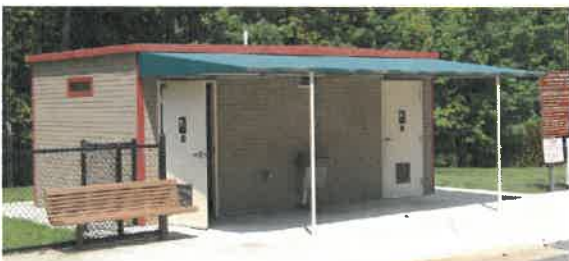
Precast Easi-Brick™ Walls, Precast Tapered Roof
