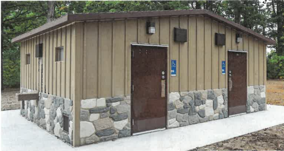
Precast Stone and Board & Batten Walls, Precast Cedar Shake Gable Roof
