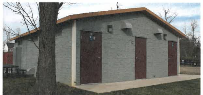
Precast Split Block Walls, Precast Cedar Shake Gable Roof
