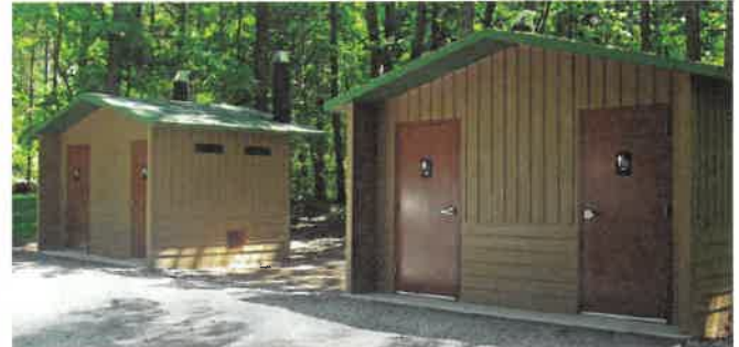
Precast Clapboard and Board & Batten Walls, Precast Cedar Shake Gable Roof
