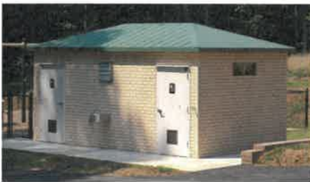
Precast Easi-Brick™ Walls, Precast Faux Metal Hip Roof
