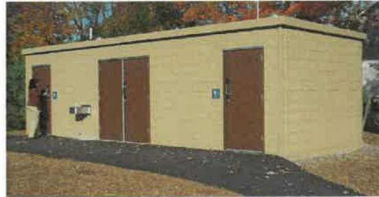
Precast Split Block Walls, Precast Tapered Roof
