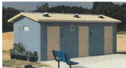
Precast Clapboard Walls, Precast Faux Metal Gable Roof
