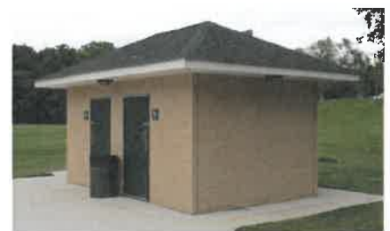
Precast Split Block Walls, Precast Flat Roof under Traditional Wood Frame & Shingles
