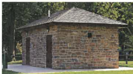
Precast Walls with Stone Veneer, Precast Flat Roof under Traditional Wood Frame & Shingles
