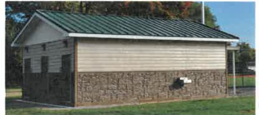
Precast Clapboard and Stone Walls, Precast Flat Roof under Traditional Wood Frame & Metal
