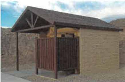
Precast Split Block Walls, Precast Cedar Shake Gable Roof
