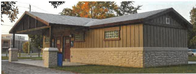
Precast Stone and Board & Batten Walls, Precast Faux Metal Multi-Gabled Roof
