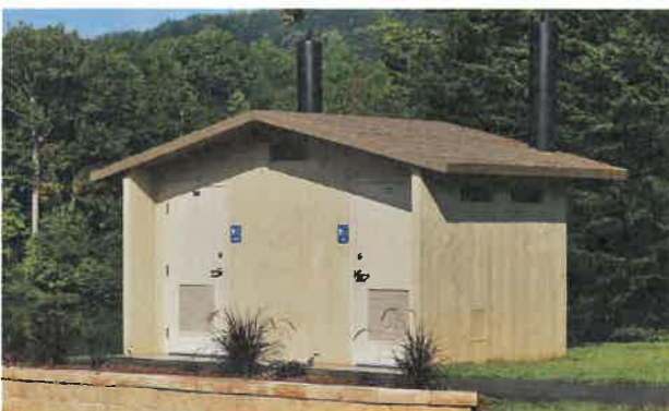
Precast Barnboard Walls, Precast Cedar Shake Gable Roof
