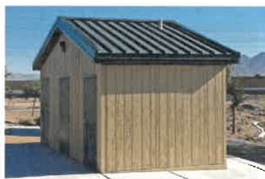
Precast Barnboard Walls, Precast Gable Roof covered with Metal
