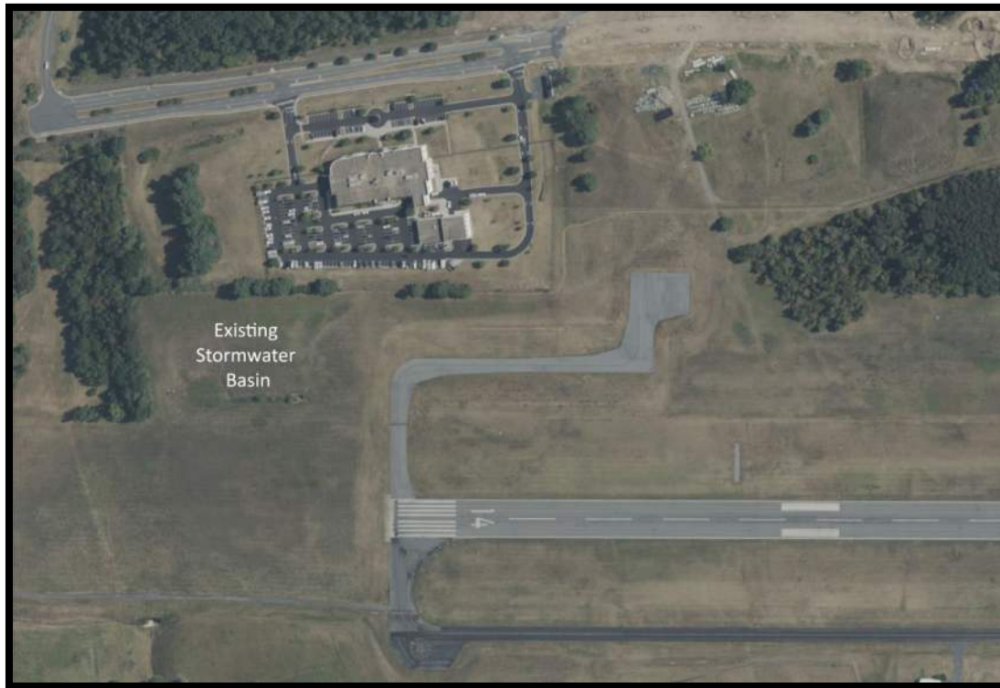
Figure 14: Existing Stormwater Basin
