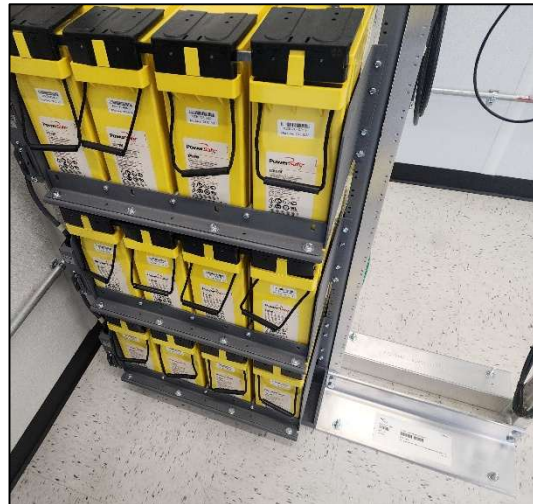
Installation of Battery Power System
