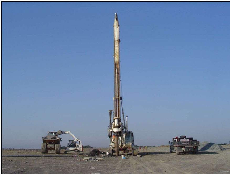
Contractor installing a gas collection well to provide landfill gas to the Gas to Energy Plant
