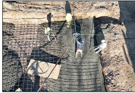
Gainesboro Tower Foundation Rebar Installed
